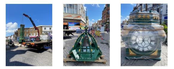
On 17<sup>th</sup> May Smith of Derby arranged for a subcontractor to erect scaffolding around the bottom two sections to enable to clock face section and capping section with the bell to be installed safely. The clock face section followed by the capping section were then lifted into place while being witnessed by the Mayor, Cllr Bonney and Ward members.
