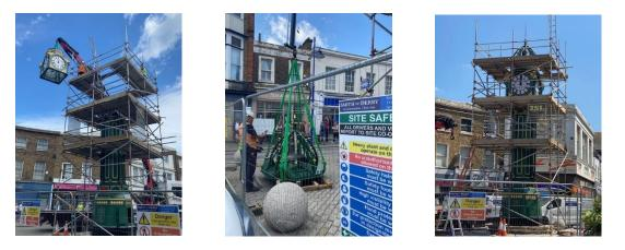
On 18<sup>th</sup> May with the tower fully in position Smith of Derby started to install the four bracket arms and new lanterns before the scaffolding was then removed. Smith of Derby also started to install the electrical cables within the tower. UK Power Networks (UKPN) were also on site to reconnect the power supply to the tower.
